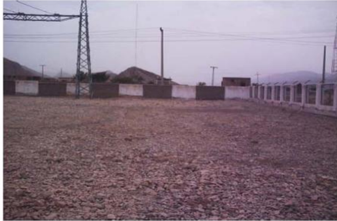
Open space at Khudkocha Grid Station
